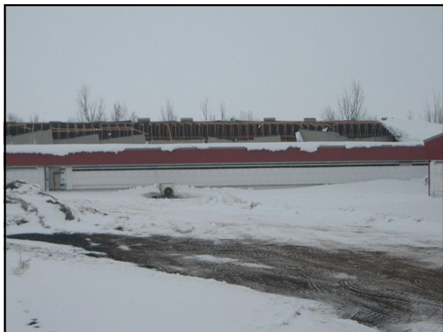
Exterior photo of collapsed hog barn
