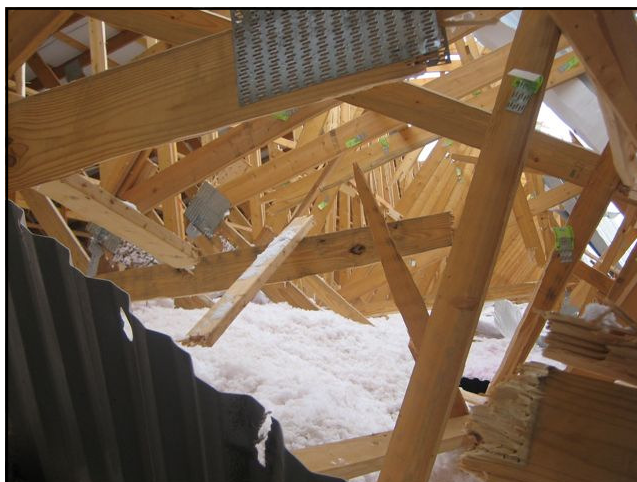
Interior photo of broken trusses of collapsed hog barn
